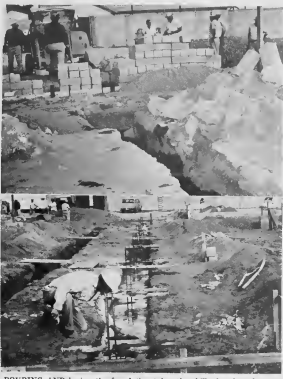
POLING AND laying the foundation takes the skill of real craftsmen.
